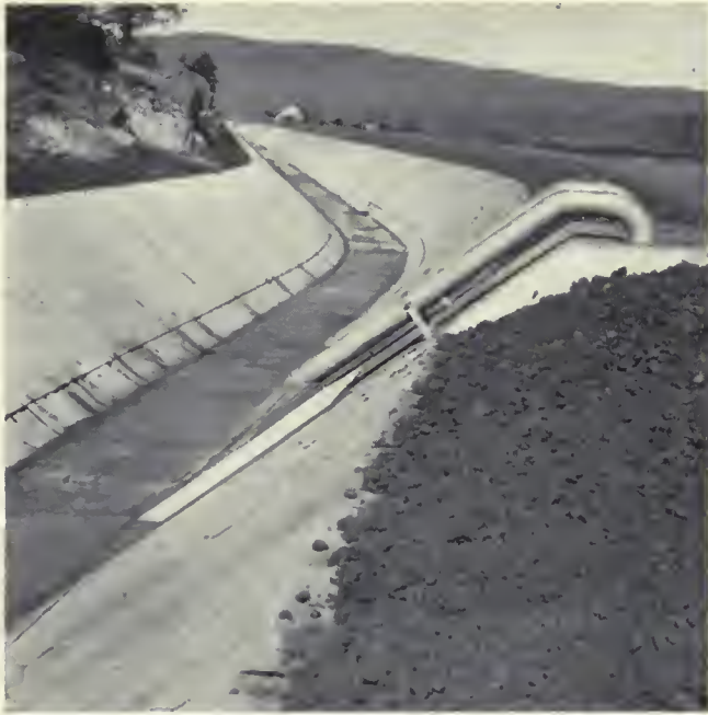
BEWARE OF THE VACUUM! —At left, note the rectangular opening in front of the pipes. When water in Colorado-Big Thompson Horsetooth Feeder Canal rises above normal, the siphon spillway goes into automatic operation, and a vacuum, strong enough to suck a man into the spillway, is created. Above, currents around check structures (like this one on the Sunnyside Canal Yokimo project, Wash.) are extremely dangerous. Photo of left by A. E. Thompson, above by S. T. Larsen.
